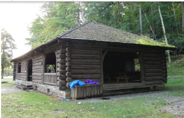
CCC Pavilion-Before. Photo by Kate M. Kocyba
