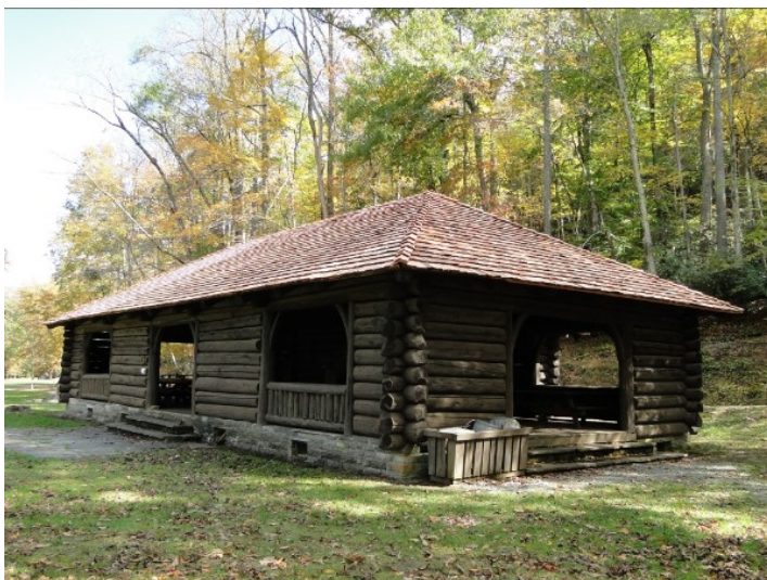
CCC Pavilion-After. Photo by Kate M. Kocyba
